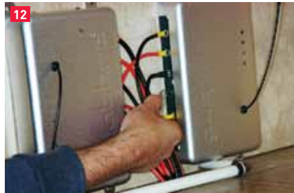
(12) With the control units securely mounted to the wall, the wires are connected to their respective terminals. (13) The kit includes split-loom conduit that is used to protect all the wiring.
